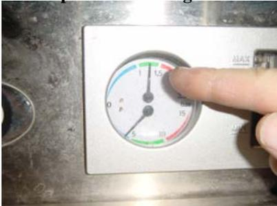
Your steam pressure gauge should read in the green zone between 1-1.4 bar. Normal operation will be 1.2 bar.
