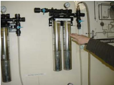
Please check the water system for replacement. Please understand when replacement should be scheduled, and talk it over with your customer. Also please check the water hardness using a test strip. The hardness should not exceed 3 grains per gallon.
