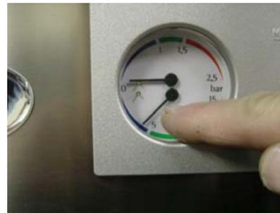
Standing line pressure should range between 3 and 5 bars of pressure. If pressure exceeds 5 bar, a pressure regulator will need to be installed. Less than 2 bar of pressure will require external pump system .
