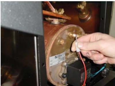
This picture is showing the level probe on the right side of the tank. Picture 2 is showing the auto fill valve. To test this function, pull the wire of the fill probe. The pump should kick on with auto fill valve. Also watch the sight glass for a change in level. The fill probe should be removed for inspection and cleaning to ensure proper water level and function.
