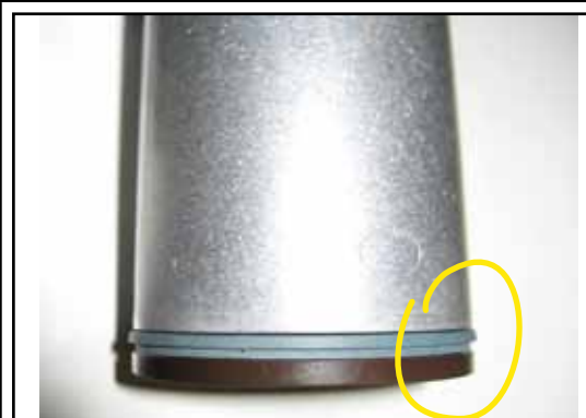
fig. 12: assemble gaskets
